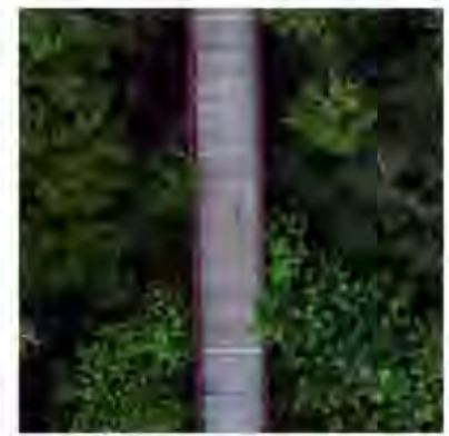
Aerial view of bridge on THT in Boydton
