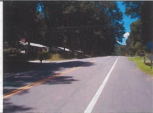
**Shared Roadway—Wide Outside Lane**—outside vehicle travel lanes that provide adequate width for both motor vehicle and bicycle travel.
